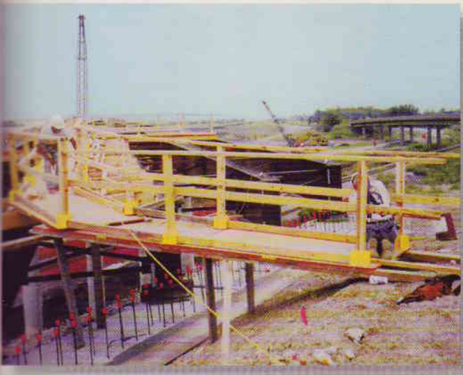
The Safety Boot Railing System is utilised on a freeway overpass
